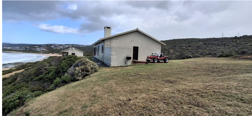
Photograph 1: Building 3 (foreground) and the existing dwelling cluster, viewed from the coastal terrace
