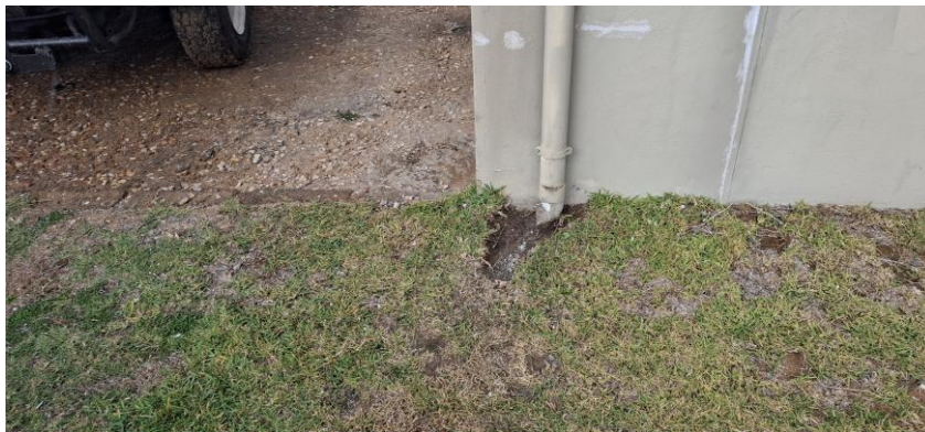
Photograph 5: Stormwater downpipe detail at the base of Building 3, relevant to erosion and dune-stability management
