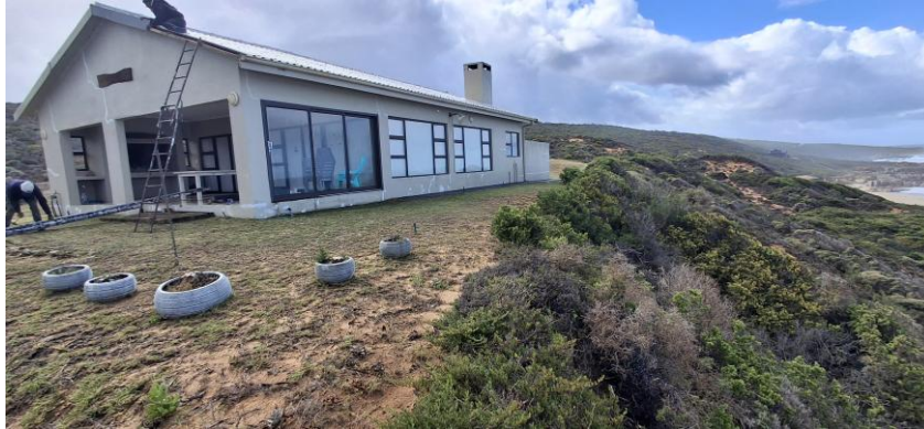
Photograph 4: Roof works to Building 3 in progress, confirming the development is confined to the existing disturbed footprint
